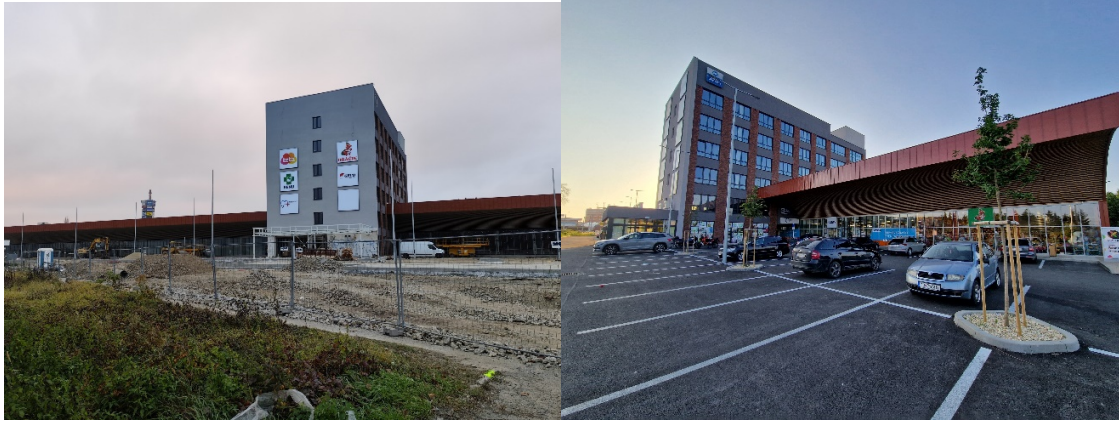
Fig. no. 3: Rebuilding of the ZPA Křížik factory (Left October 2024, right June 2025).
