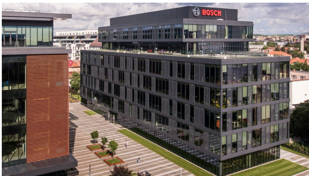
Figure 1. Bosch Engineering Center , Cluj-Napoca, 2020 ©Bosch Engineering GMBH
