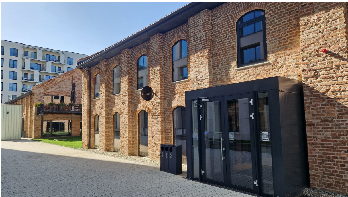
Figure 3. Stables co-working spaces, Cluj-Napoca, 2023
