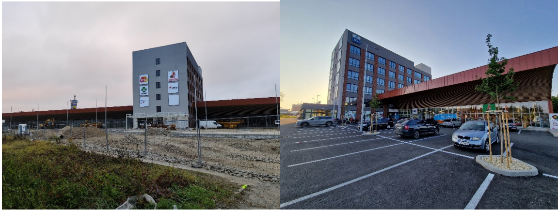
Fig. no. 3: Rebuilding of the ŽPA Křížik factory (Left October 2024, right June 2025).
